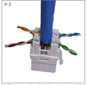
2. Place the wires into the slots according to the wire scheme.
